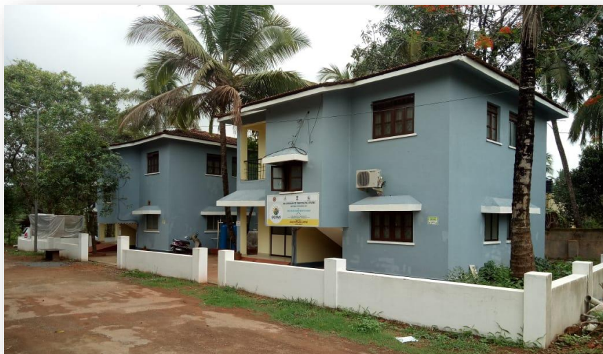
MPC at Pontemol-Curchorem
